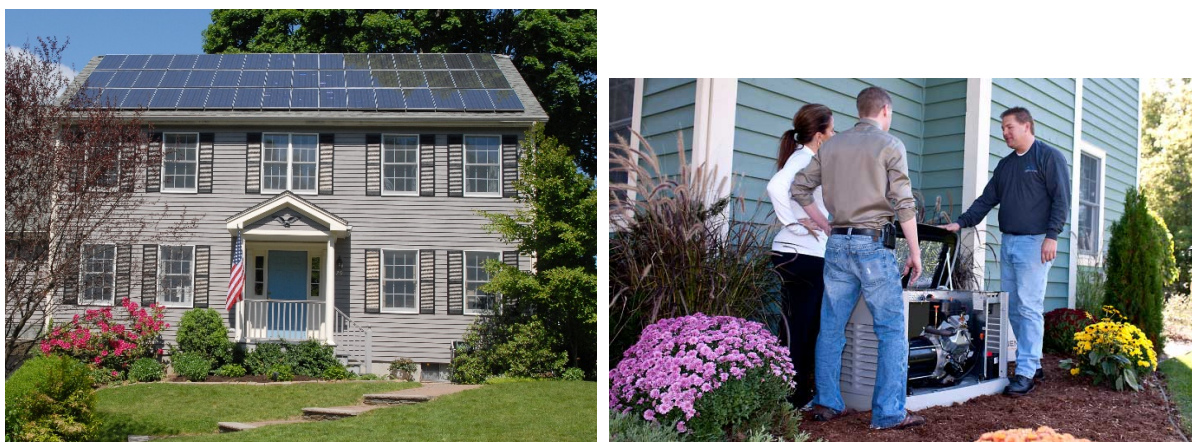
Figure 6. Left: solar panels on roof. Right: a 21 kW standby generator (Generac, Guardian model).
